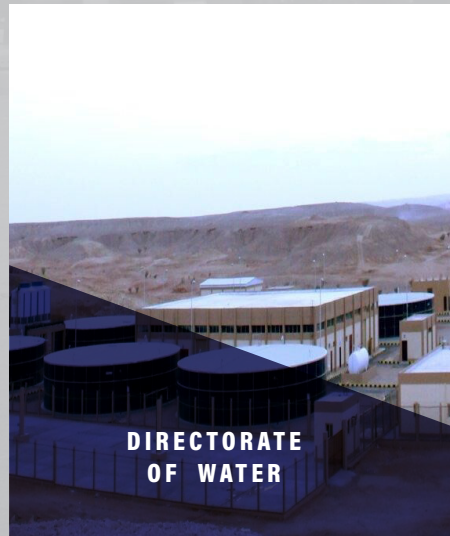
Sulayyil Reverse Osmosis plant 10,000 m3/d
