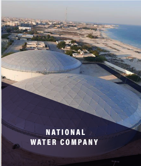
50,000 m3 Welded Steel Tanks in Al Khafji
